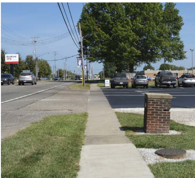
IMAGE 2-3: SR44 Sidewalk Conditions
