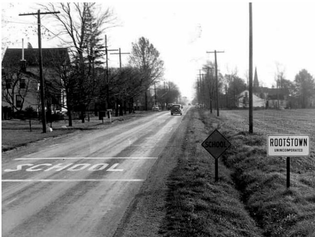
IMAGE 2-1: State Route 44 Looking South
